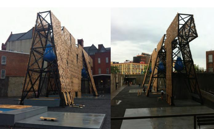
scraps, which functions as a giant aqueduct. Built in 2013, *Party Wall* is intricately designed such that certain panels in the structure can be detached and used as benches, communal tables, and a series of small-scale performance stages. The piece provides shelter and shade while still functioning as a demarcating "wall."
